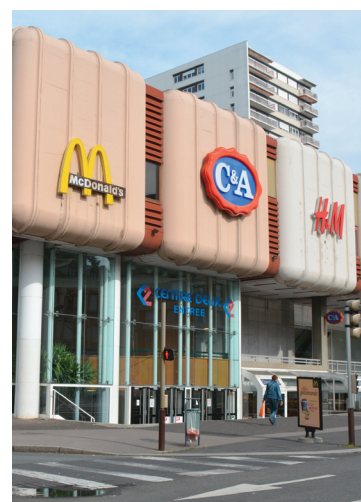
Centre commercial Centre 2
